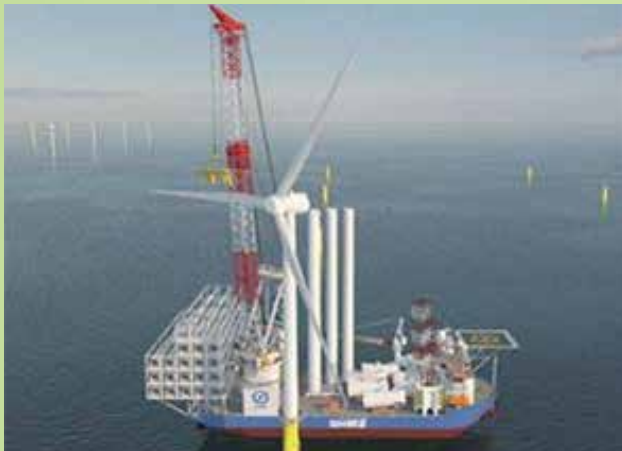
SEP vessel attaching blades
