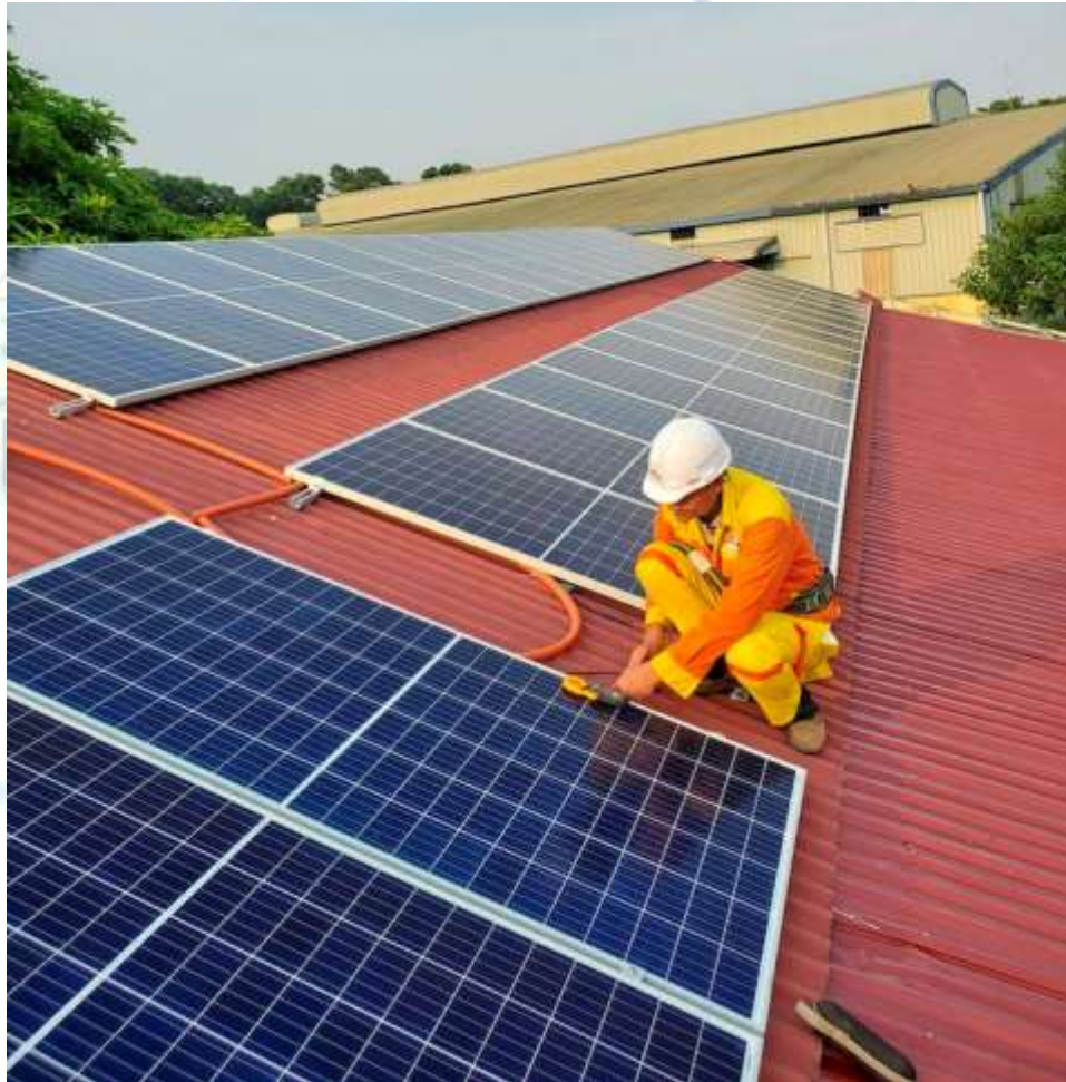
Image 1: Man installing solar panels on a roof, Pexels
