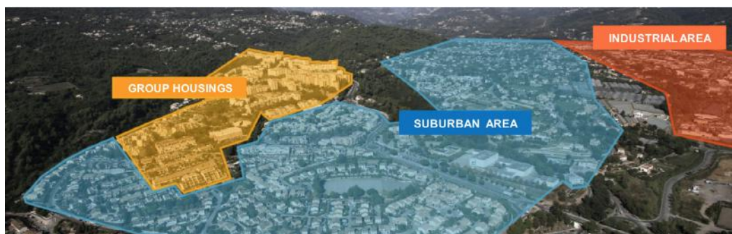
Figure 3-3 Microgrid site at Carros Source: Nice Grid 12
