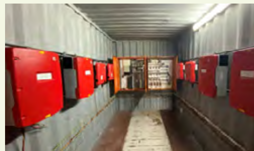
Solar PV Power Inverter Banks
