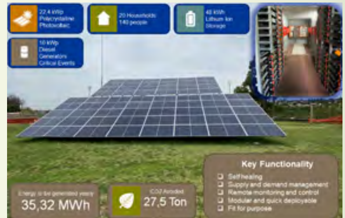
Figure 2: Modular Containerised Microgrid
